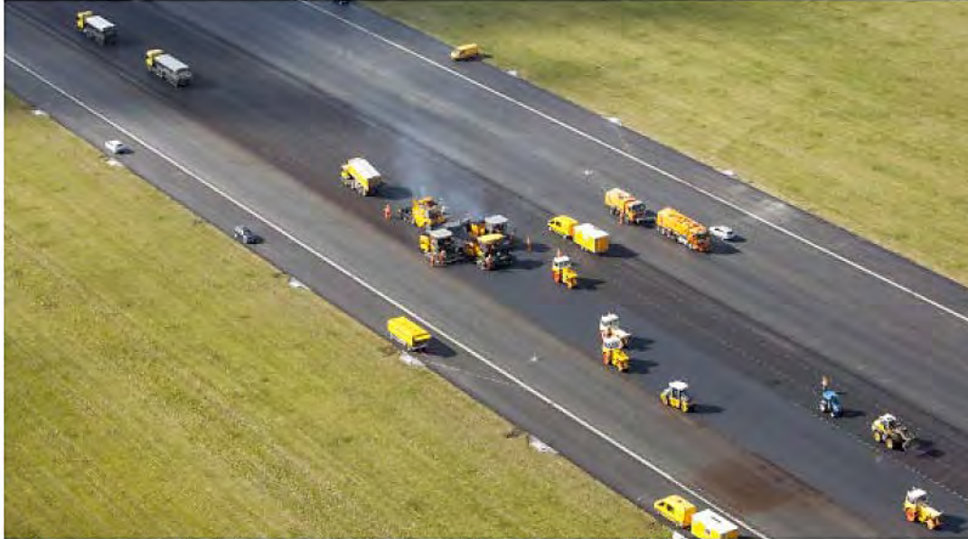
Heijmans paving the Polderbaan with Cargill's Anova® Rejuvenator. © 2021 Heijmans
