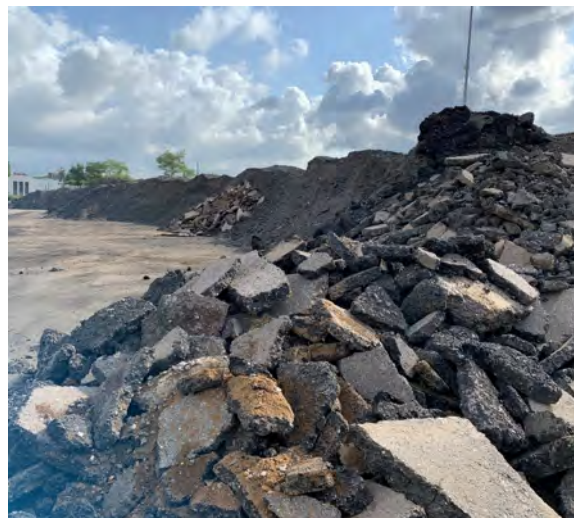
(picture: Federal Highway Research Institute, Kalantari)
